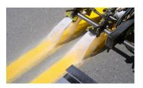
The retro-reflective properties of the Glass Beads cause the road marking paint to light up and become brighter as the light beams from the vehicles' headlights falls on it
